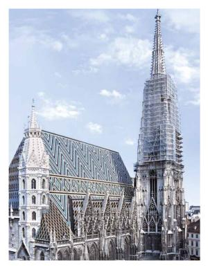
We used a bespoke modular scaffolding system for St. Stephen's Cathedral in Vienna which was erected around the building without the use of anchors
